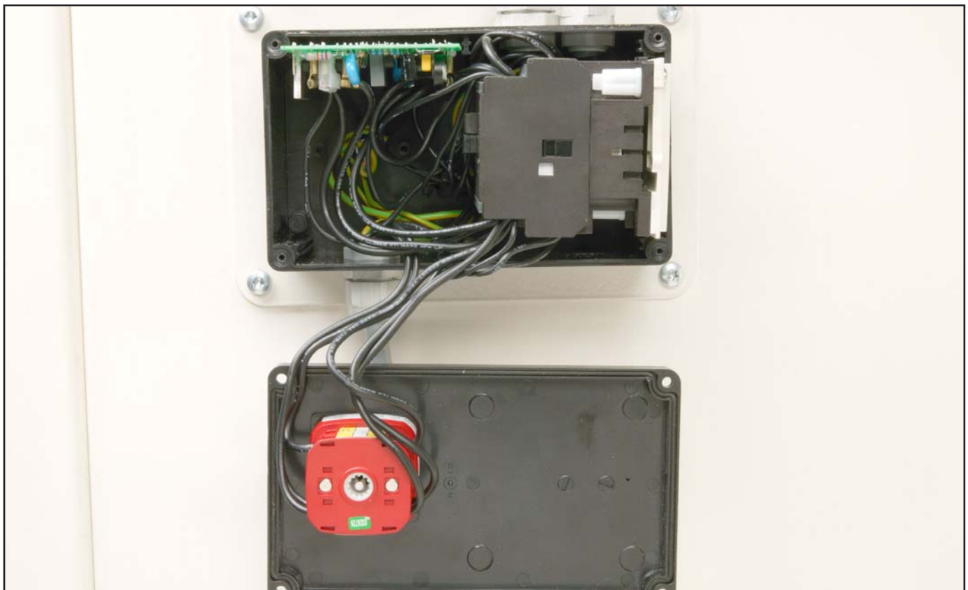
Figure 101. Main switch box wiring.
